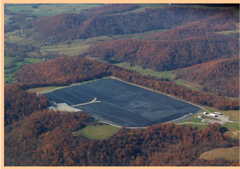
2006 aerial photo taken from the northeast
