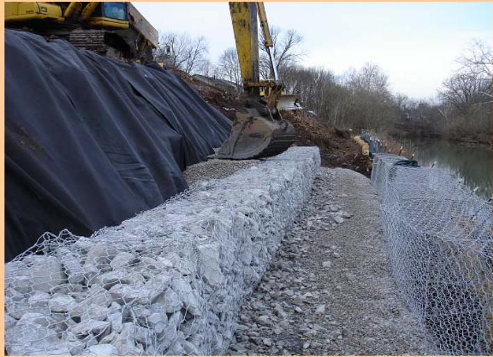
Above: A gabion structure stabilizes the banks of the Elkhorn Creek at the Briar Hill landfill, Scott County.
